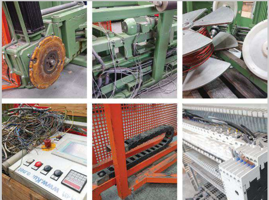
Close-ups of the retrofit system before the conversion.
